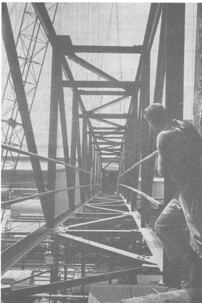
SYRUP BRIDGE —Structural steel bridge is placed to span gap between Syrup Refinery and Syrup Packing House during expansion activity this month. Bridge will carry sweeteners from processing to loading for shipment to Staley customers. Additional track and cooling facilities are also being built to accommodate increasing number of orders for Staley corn sweeteners.
