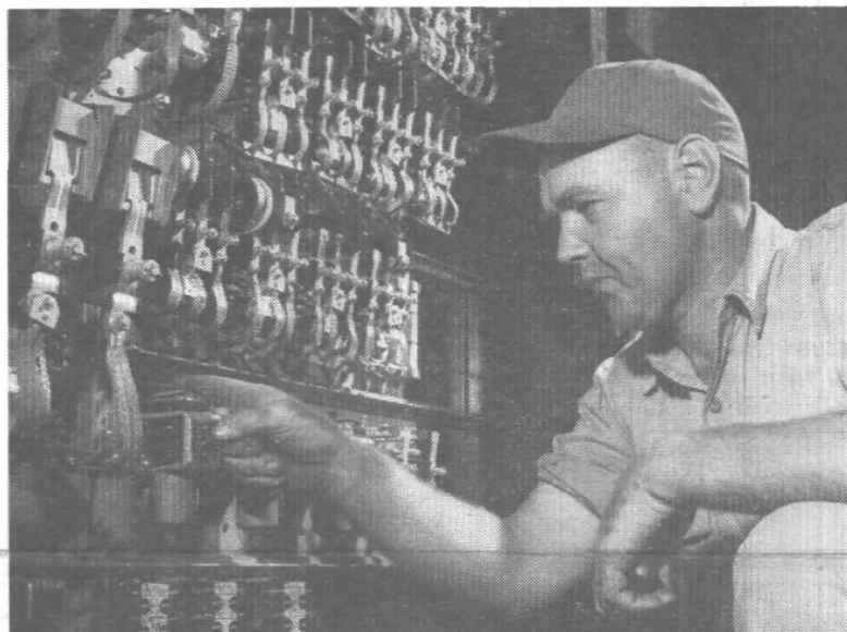
INSTALLING electronic controls for first of three new elevators for Administration Building, Arthur Kramer of Otis Elevator Co. checks intricate connections in automatic control system.
