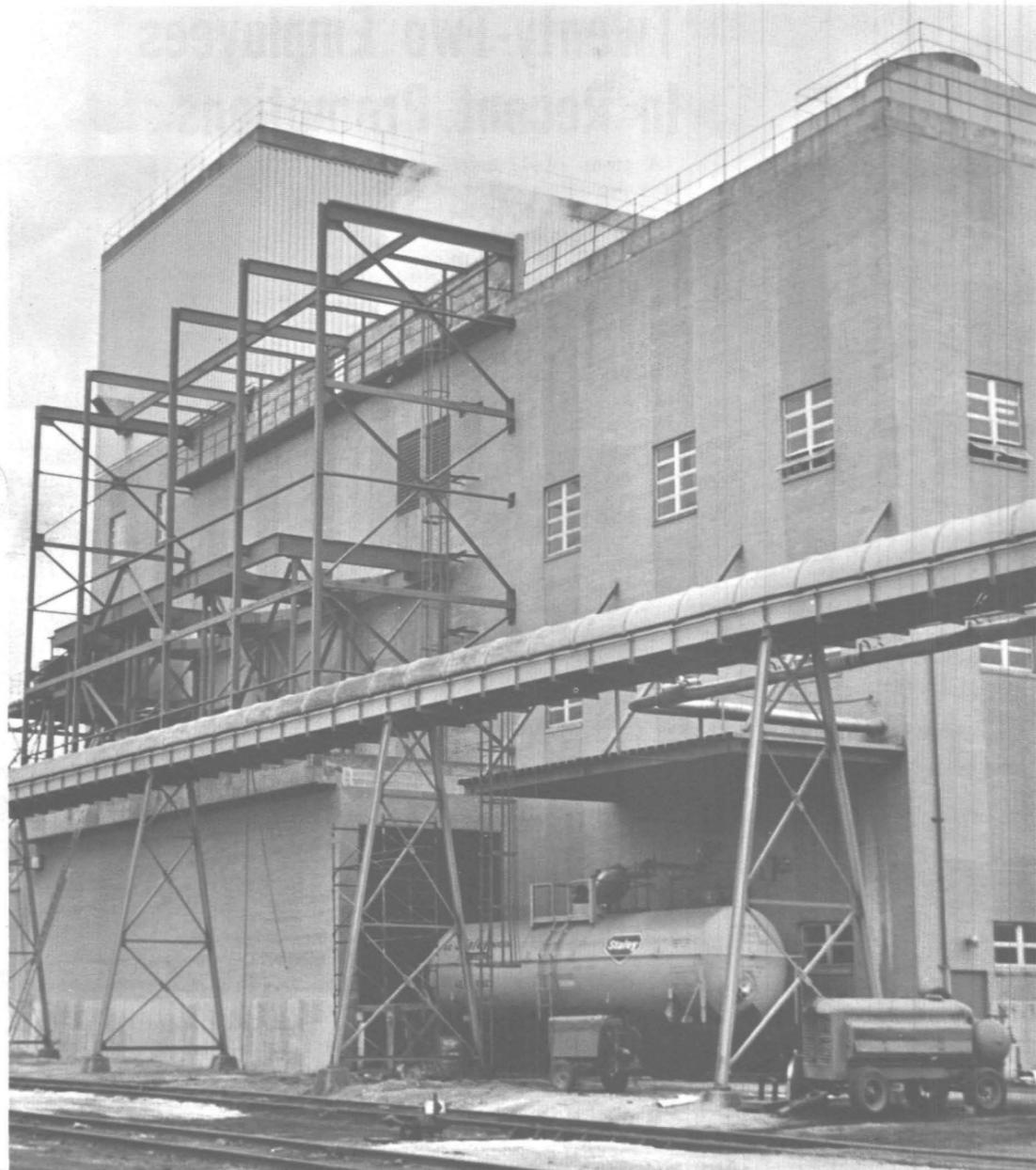
**DEXTRROSE STORAGE FACILITY PROGRESSING**—Steelwork has been erected for a dextrose bulk storage facility on the north side of 44 Building that will enable faster, more efficient loading of hopper railcars and truck trucks. The structure will house three large holding tanks for dextrose waiting for shipment in bulk quantities.
