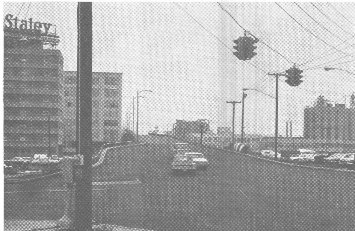
NEW LOOK FOR STALEY VIADUCT —This is how the 22nd Street intersection and Staley viaduct looked after expansion work and black-topping were completed, providing greater ease
