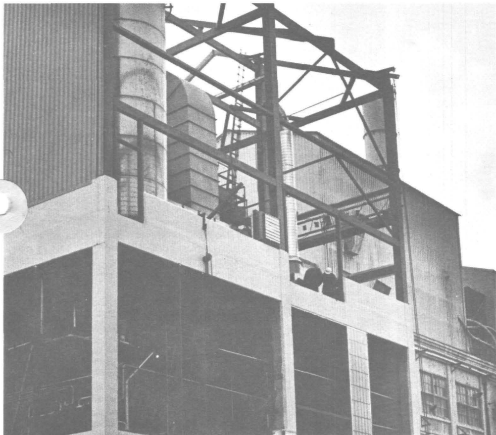
Construction progresses on the multi-million dollar expansion for the flash drying capabilities at Decatur Plant. Startup is expected in January.
