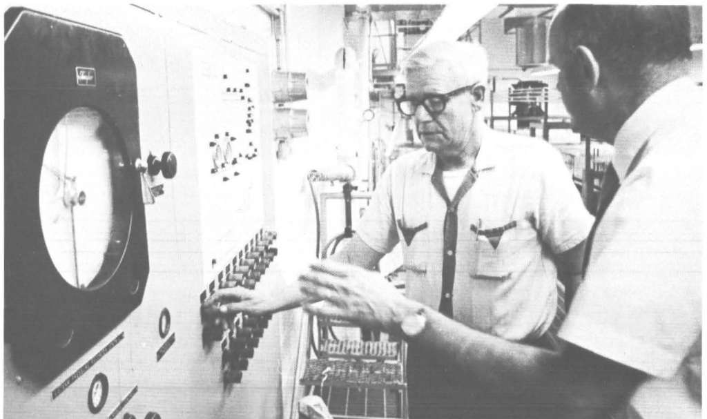
Command central for the new process is this electronic panel board. Operator Bernard Runyen and process design engineer Bruce Dwiggins review operating instructions.
