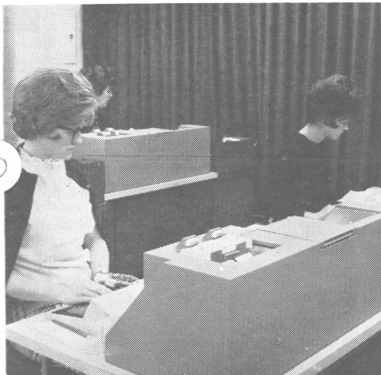
Shirley Morse, Marna Caldwell and Sondra Simpson, keyed data equipment operators from left, convert source documents to punchcards on keyed data machines. Information can also be converted to magnetic tapes.
