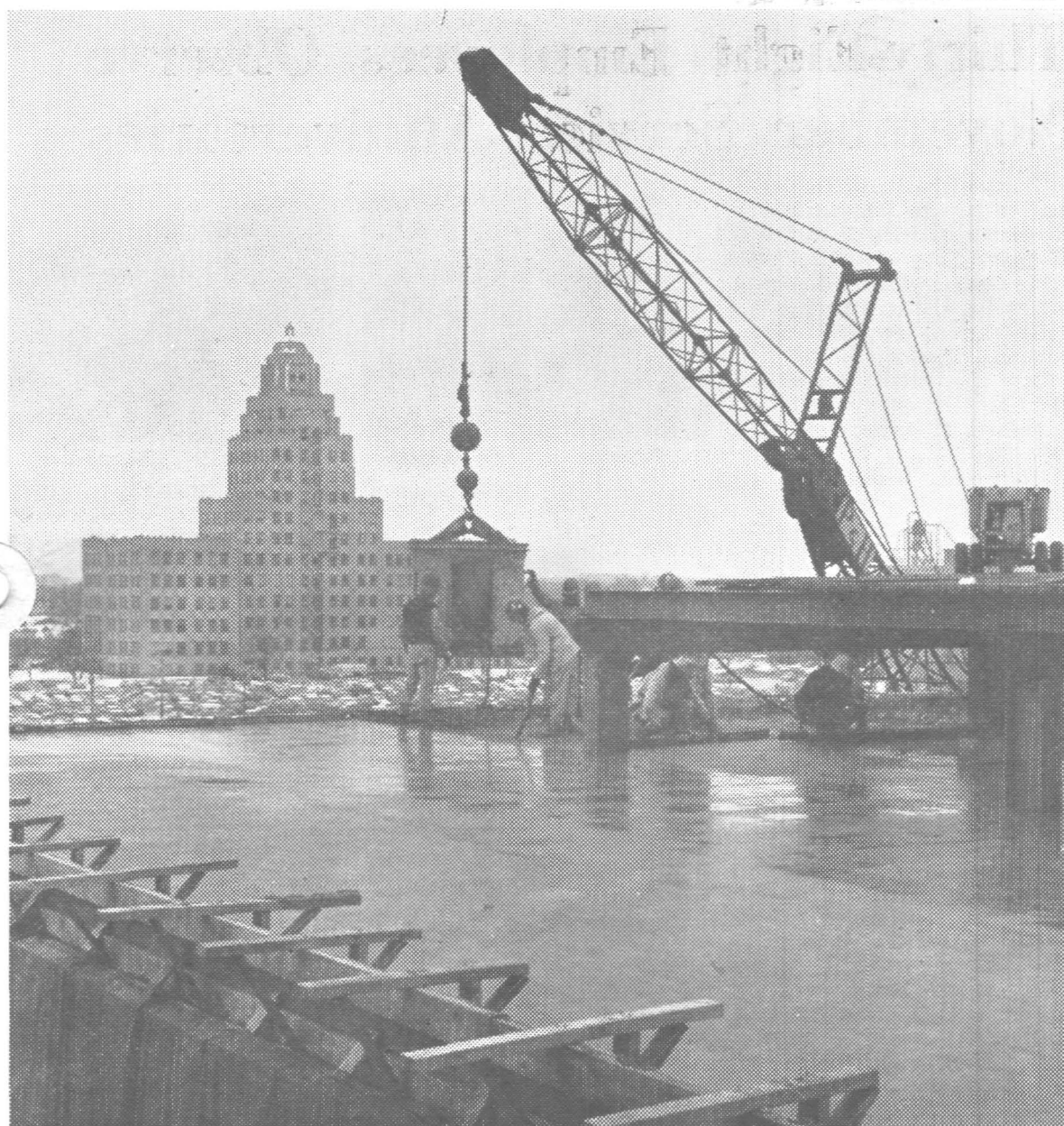
PROCESS BUILDING ROOF POURED —Roof of the new process building addition to the Dextrose Plant is poured and finished, by workmen. Steel framework at right will support a cooling
