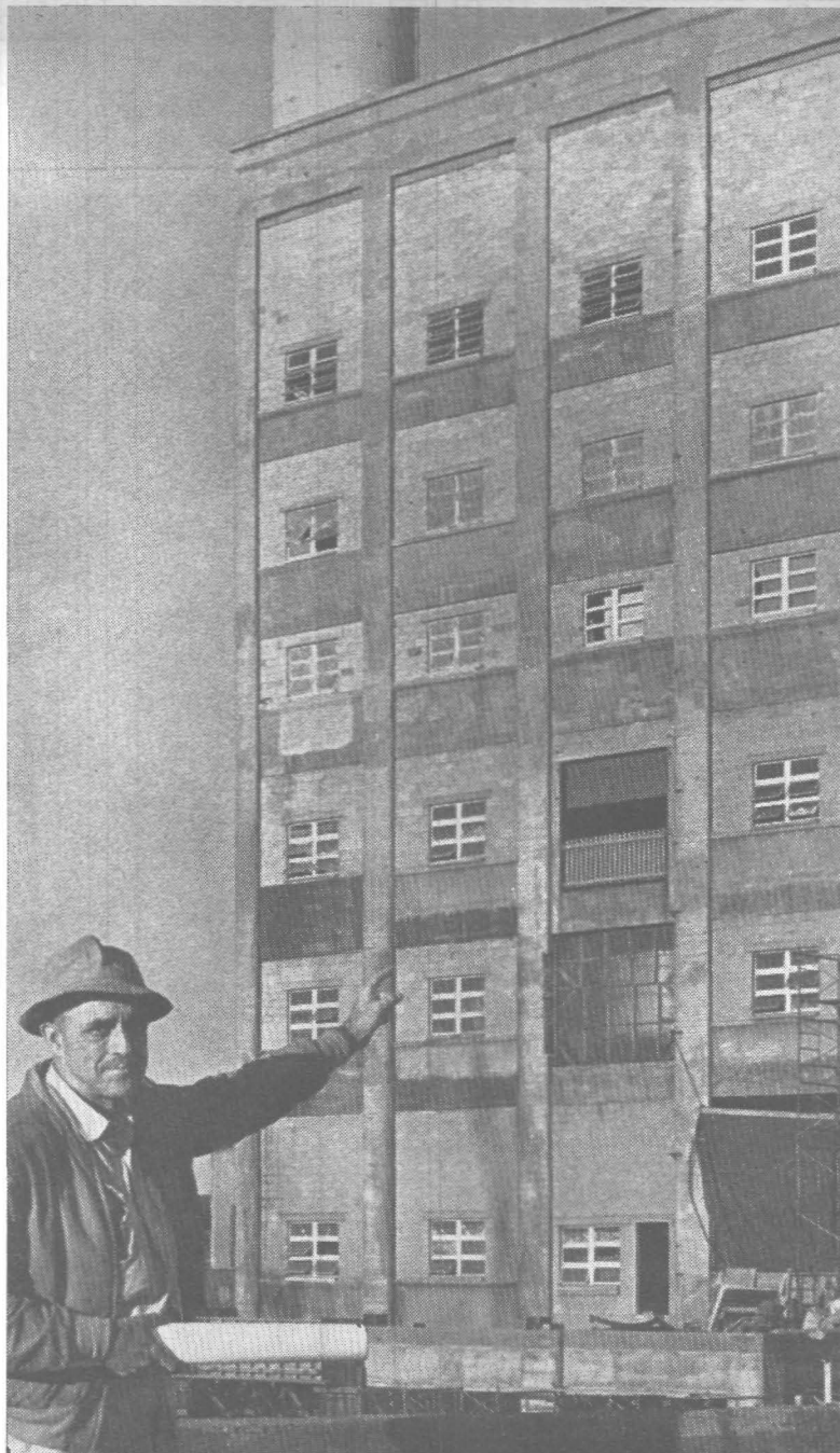
NEW LOOK—Construction engineer Jack Grant points out new aluminum-sashed windows on west section of 10 Bldg. Two-year replacement project is in final stages of completion.
