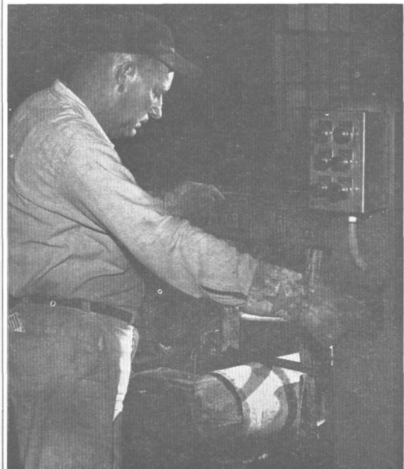
Melvin Workman threads a pipe for use at the Syrup Refinery as a cutting length.
