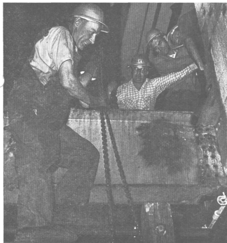
Riggers remove a structural steel beam to get an old bone filter out of the Syrup Refinery. From left, Orville Hinton, lead man; Alvin Morris, Richard Karl and Ronald Devore.
