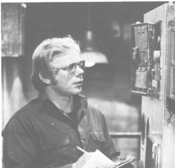
Mike Blackwell, upper left, makes a reading on the Parkson stripper which removes residual monomers from the polydene. Mike is an operator.
