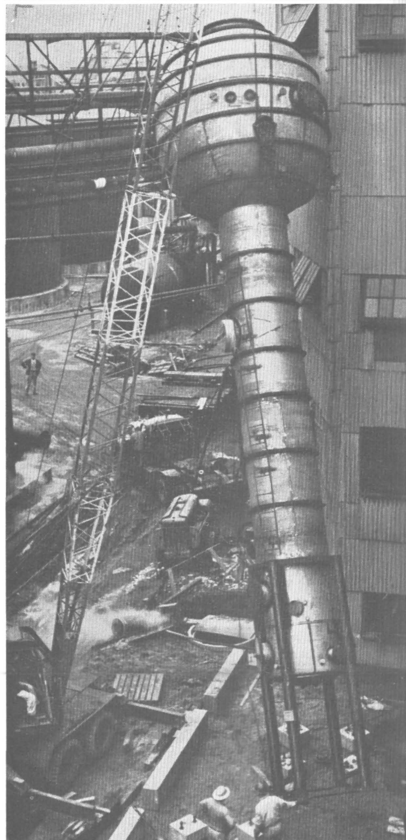
CLOSE SHAVE —A bit too close, in fact, as some corner stripping on the Feed House wall was shaved off by this giant evaporator stage passing on its tedious path to rest on concrete footings. Workmen succeeded in guiding the 51,000-pound stainless steel structure, along with two others slightly smaller, to resting places in the area soon to be enclosed as the Feed House addition. The wall seen here will be expanded around the new installation.
