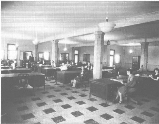
This Is How a Wing Looked in New Admin Building in 1930 In Those Days It Was One of the Most Modern in Decatur
