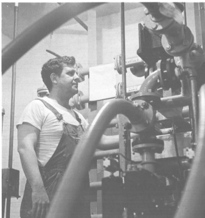
Jim Rethinger Selects the Chemical for a Reactor The Quantity of Chemical Is Controlled Automatically
