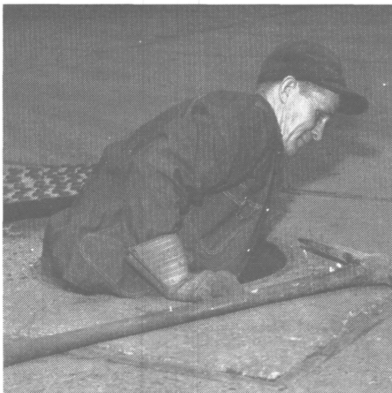
ROOM TO SPARE —Frank Russell, rigger leadman, Yards, has room to spare as he climbs down a manhole to take care of some repair work. A majority of Staley employes physically get down to work every day. Maintenance employes are among the most active in this respect.
