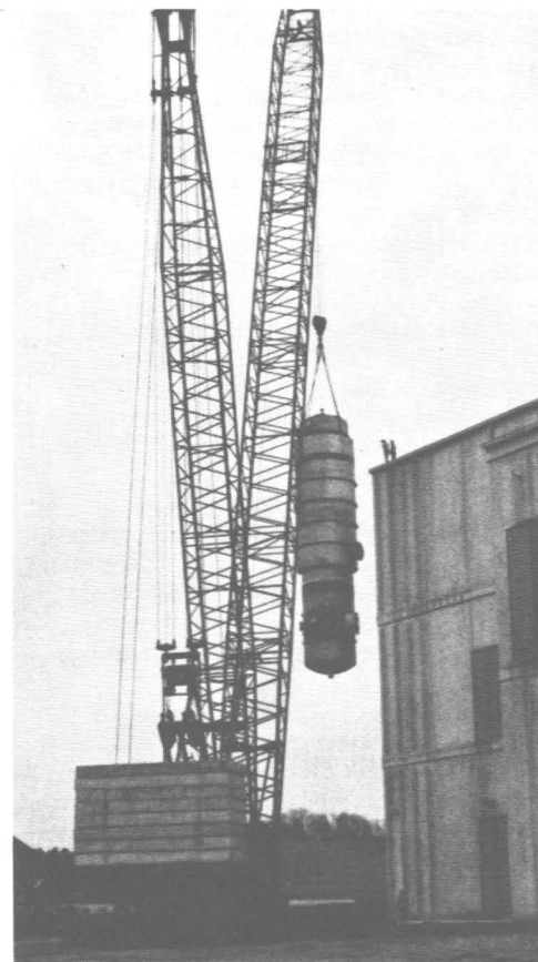
Two cranes prepare to lift the evaporator steam chest from the rail car bed and take it to the roof of the Loudon refinery through which the large vessel was put in place. A section of the roof is removable, making this operation feasible.
