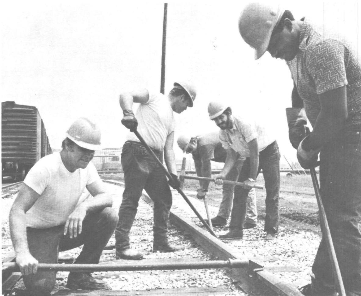
Laying track for railroads is, as it has always been, a job requiring the skills of people. Working on this section are, left to right, Tom Brabender, Larry Miller, Bob Kelly, Tom Roberts and Willie Green.
