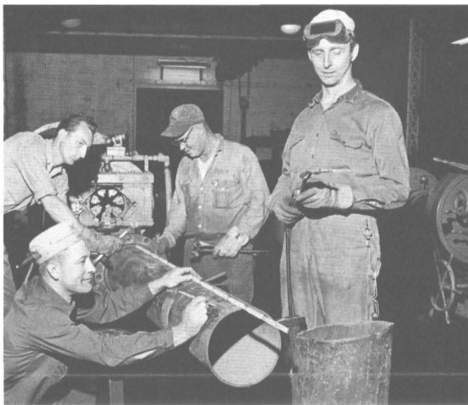
Dale Born Measures Replacement for Ruptured Line Assisting Are (L-R) Max Napierski, Gil Kratzner, Don Klingler
