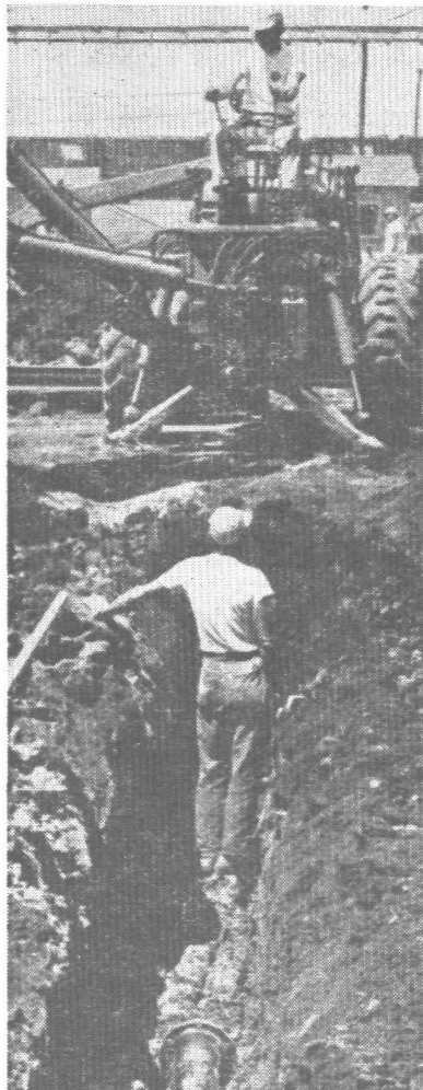
DEXTROSE DITCH —Progress on the dextrose building centers on extending pipe for sewer lines.
