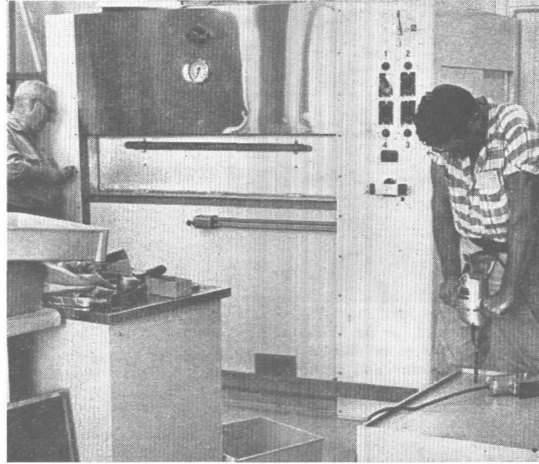
SOMETHING COOKING —Or at least it will be, in this new equipment being installed at the Research Center's experimental kitchen. Working on the new additions are Bus Coulson, left at oven, and Earl Shobe, drilling cabinet.
