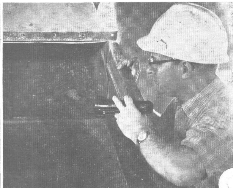
LONG-WEAR —Area Maintenance Engineer Charlie Frey shines light into Urethane-lined Mayo to demonstrate how product has stood up over 30 months.
