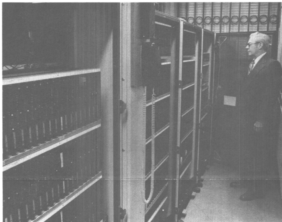
Harold Doddek looks at the Dimension 2000 switching system computer control common equipment which, besides switching, handles all of the number dialing, connections to various tie-lines and path selections. The cabinets contain circuit boards that control each line, including trunk, tie-line and station circuit boards. All of them are fused and cross connected to the memory and software of the computer.
