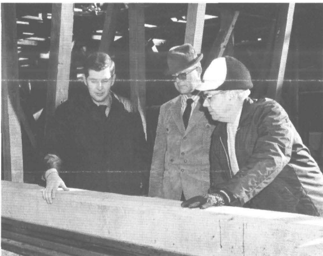
Mel Picker (L) Checks Ceilcrete Coating on Tower Basin Theron Tinker (C) and Frank Grossman Lend a Hand
