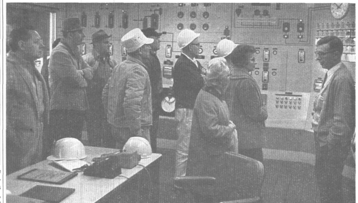
FOREMEN'S TOUR — Section Superintendent Dave Mitchell explains what the relation of the panels in the Central Control Room of the Dextrose Building are to the various processes involved in making dextrose to several foremen who participated in a tour of 44 Building last week to acquaint them with the Company's newest facilities.
