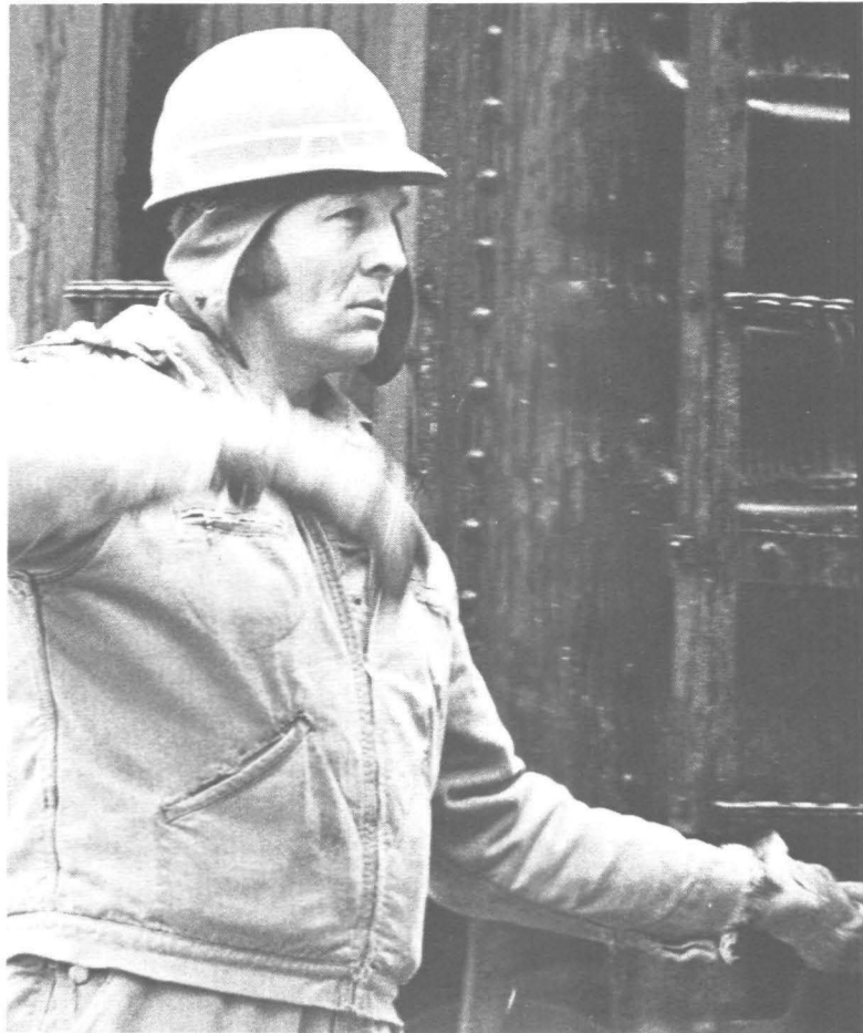
Gary Mahannah, building cleaner, guides a car from the rail car dump.
