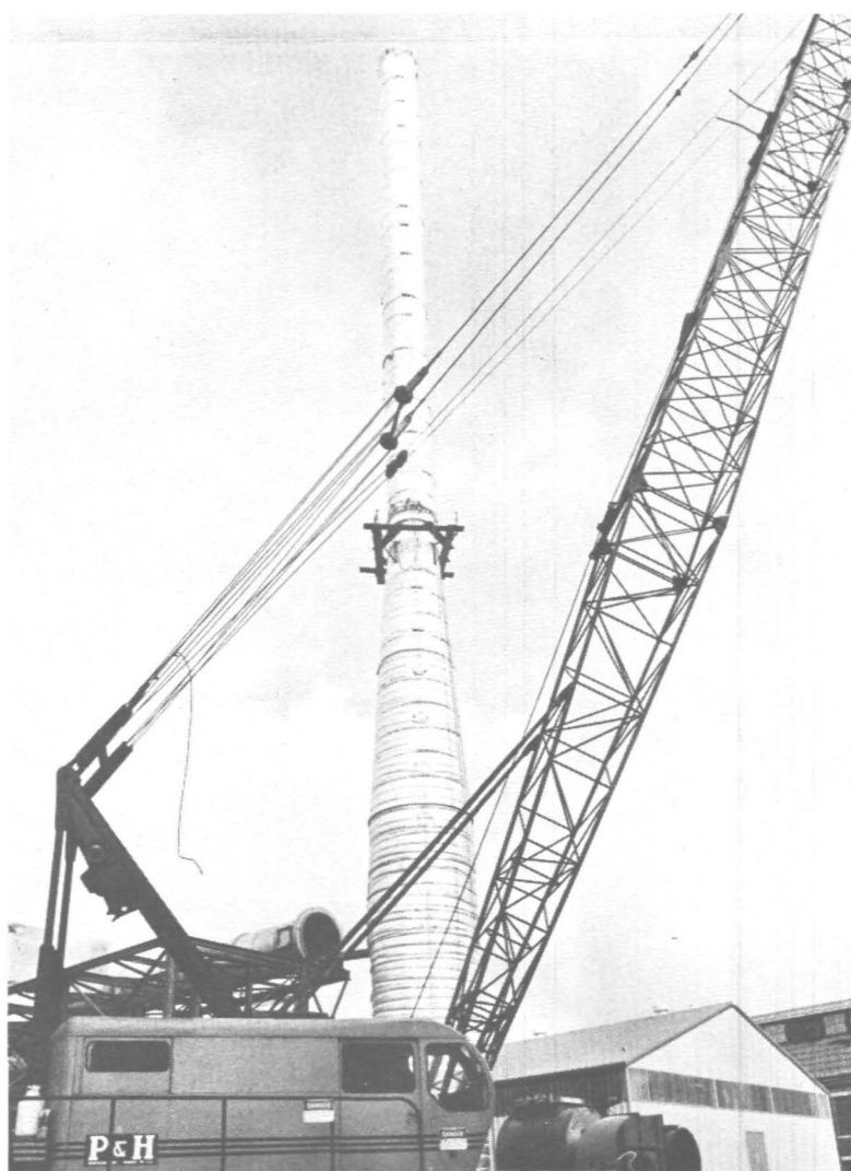
A space-age appearance was given to the Decatur plant when the new stack for 14 building was installed. The shiny material on the stack is exterior insulation which was removed when refractory insulation on the inside of the stack was installed. The stack offers a highly visible reminder of the extensive expansion throughout Staley.
