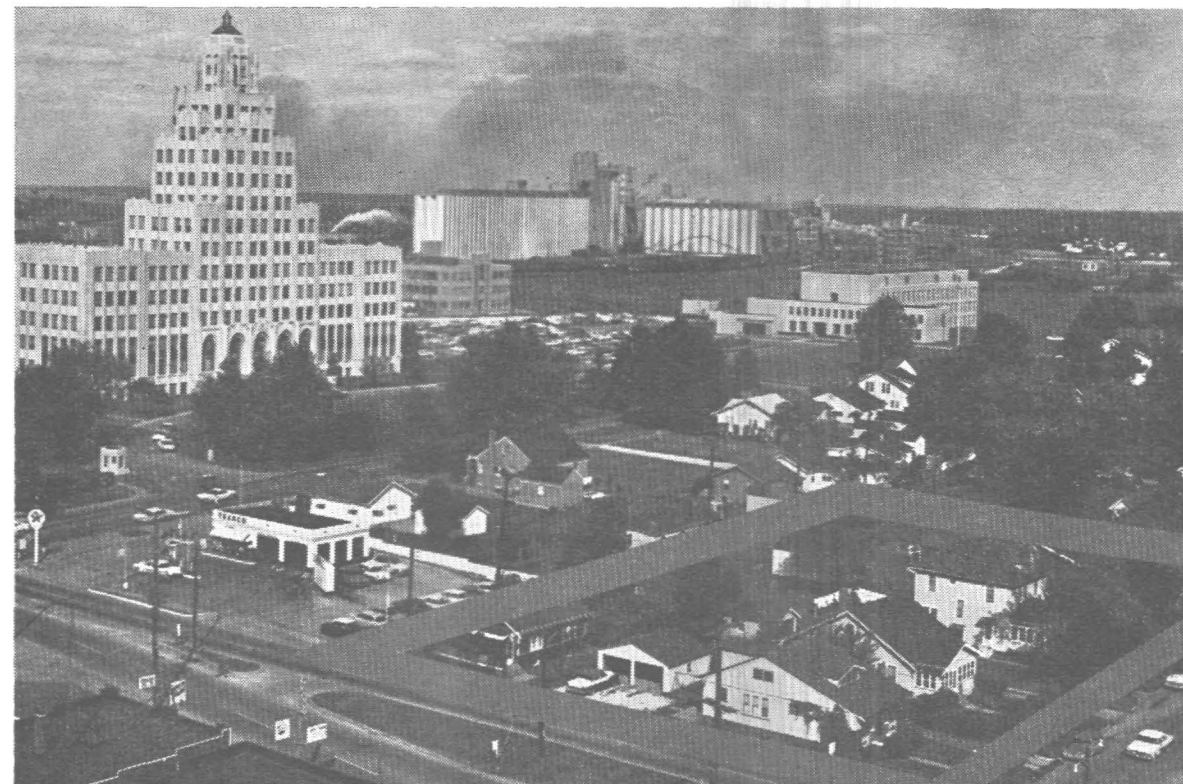
CREDIT UNION SITE —Tract on 22nd and North Sts., outlined by grey brand above, will be site of new office building to be constructed by the Staley Credit Union.
