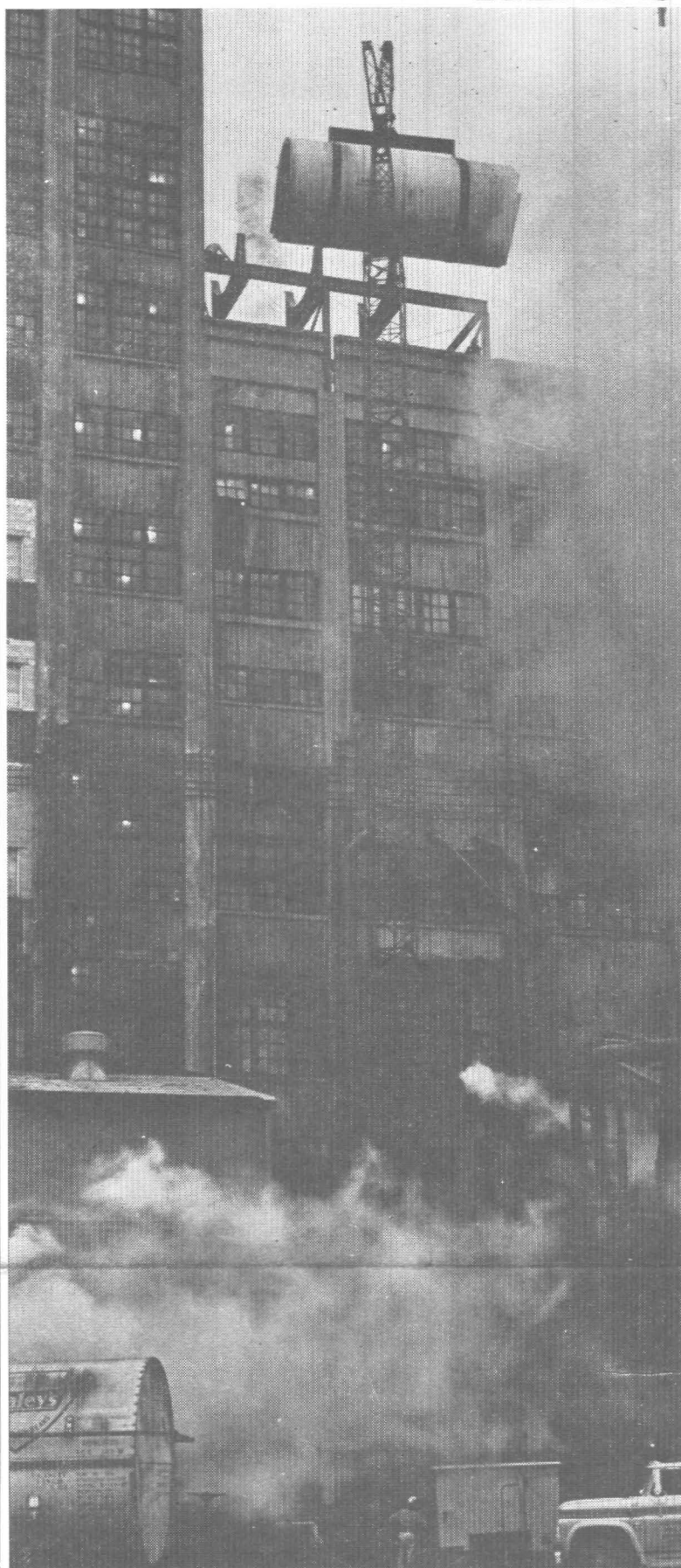
... AND OVER—Some 150 feet later, the mammoth tank is set to rest on its cradle.
