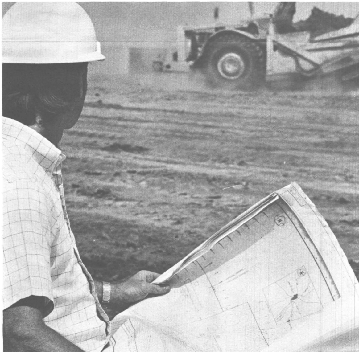
Site preparation at Lafayette is on schedule. Engineering trainee Terry Greene overlooks some of the activity which has seen more than 70,000 square yards of dirt cleared to date.
