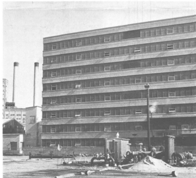
Gas Meter Is Installed But There's Not Enough Gas Boiler Conversion (Stacks in Background) Is Affected
