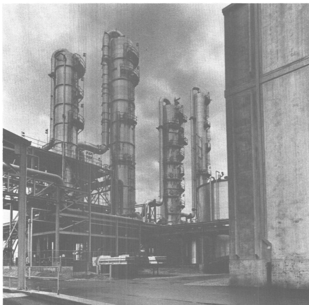
The four distillation columns, a skyline marker of the Loudon plant, concentrate alcohol from fermented material into anhydrous alcohol.
