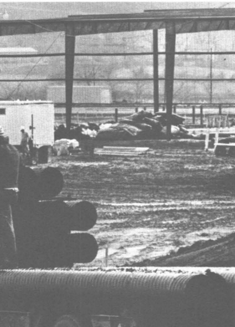
Underground piping is being unloaded at the Loudon site. In the background, structural steel is being erected for the maintenance stores building.
