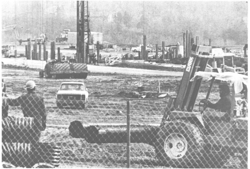
Activity is in high gear at the Loudon plant site where, in this picture, piling and a pile driver are captured in the background along with a roadway, one of the first facilities put in at the location of the company's fourth corn plant.
