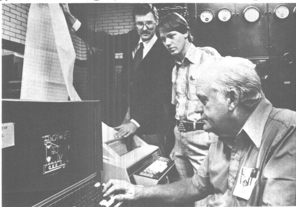
The switchboard operator in the engine room, Frank Waller, observes 24 boiler's functioning, which is controlled by the new system. At the same time, George Virgil, left, and Jeff Dehn look over utility printouts.
