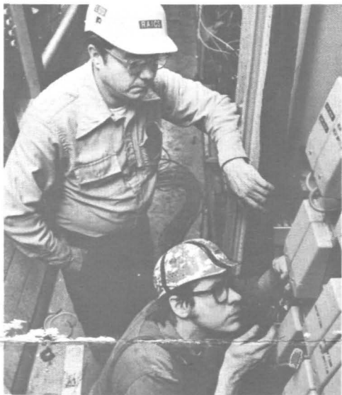
Jim Ward works on a starter in the motor control center while Lou Raics, electrical foreman, observes.
