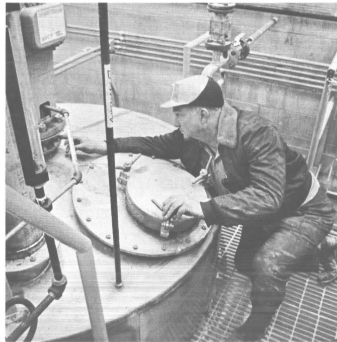
Millwright Zeke Reid Checks Out an Operation It's the Agitator on the Unit's Filter Feed Tank
