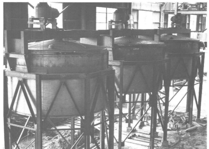
Syrup Coolers Are in Place in Syrup Refinery Awaiting Pipefitting Work by General Contractor
