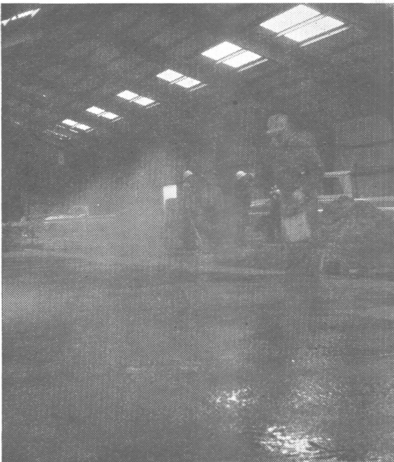
FLOOR POURED —A workman scatters cement dust over the freshly poured floor in the addition to the Black Warehouse. The 25,000-square foot addition is now virtually complete.
